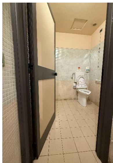
31 toilets with grab bar
